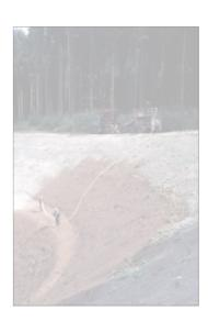
Soil stabilizer Terrafix consists of 100% active substance and is emulsified directly on site in spray equipment fitted with an agitator. The tank of the equipment is filled, in well-established manner, with the spray mixture of water, seed mixture, and mineral of organic fertilizers and with such other necessary soil auxiliaries or conditioners needed for local conditions.
